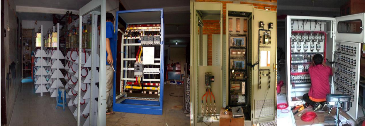
Picture 2. Electrical & Control Services
